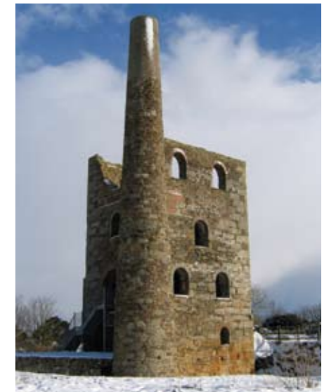
The pumping engine house at Wheal Peevor, near Redruth, Cornwall
